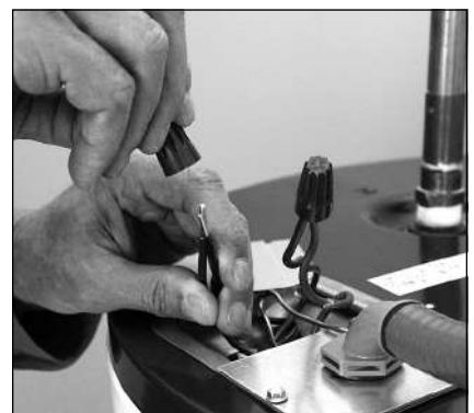
Figure 19 - Connecting the electrical wires.
