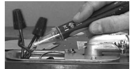
Figure 32 - Non-Contact Circuit Tester
