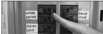
Figure 24 - Circuit Breaker
